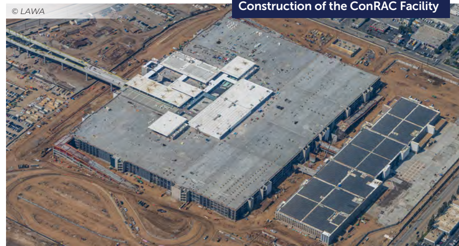
Construction of the ConRAC Facility
