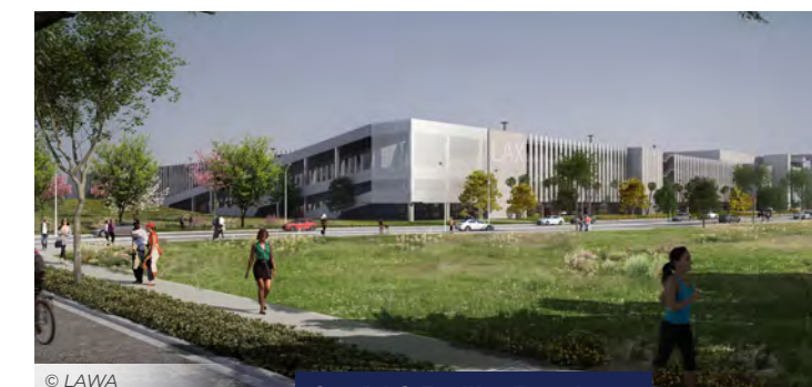
ConRAC Facility Exterior
