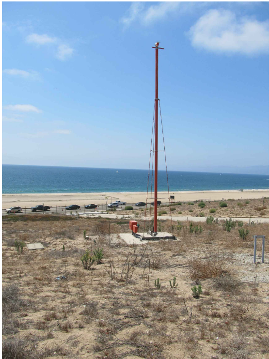
1. View of MALSR Station facing west.
