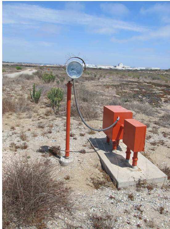
2. View of flashing Station facing east.
