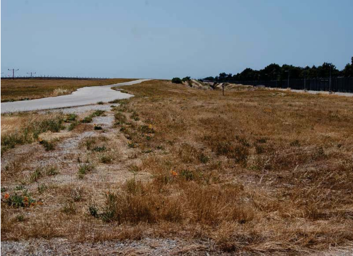
Image 2.2-1. Proposed Undertaking Area, Showing (Left to Right) Runway 6L-24R, Road Segment No. 2, the Eastern End of Argo Ditch, and the Airport Operations Area Fence, facing east
