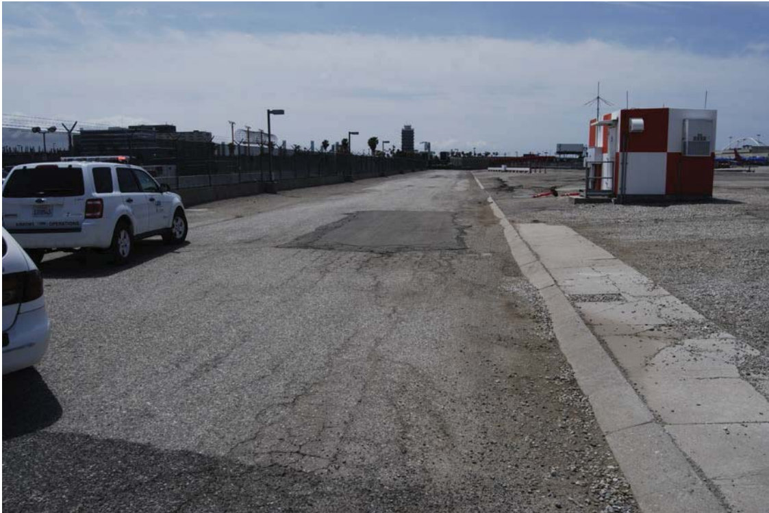
Image 2.2-3. El Manor Avenue, Located at the Eastern End of Runway 6R-24L, facing south. FAA localizer equipment (navigational aid) is housed in the structure shown in the upper right portion of the photo.
