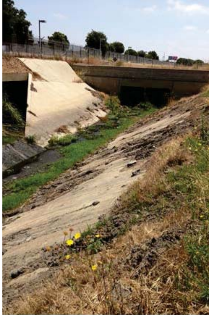
Image 5.2.1-1. East End of Argo Ditch, looking east
