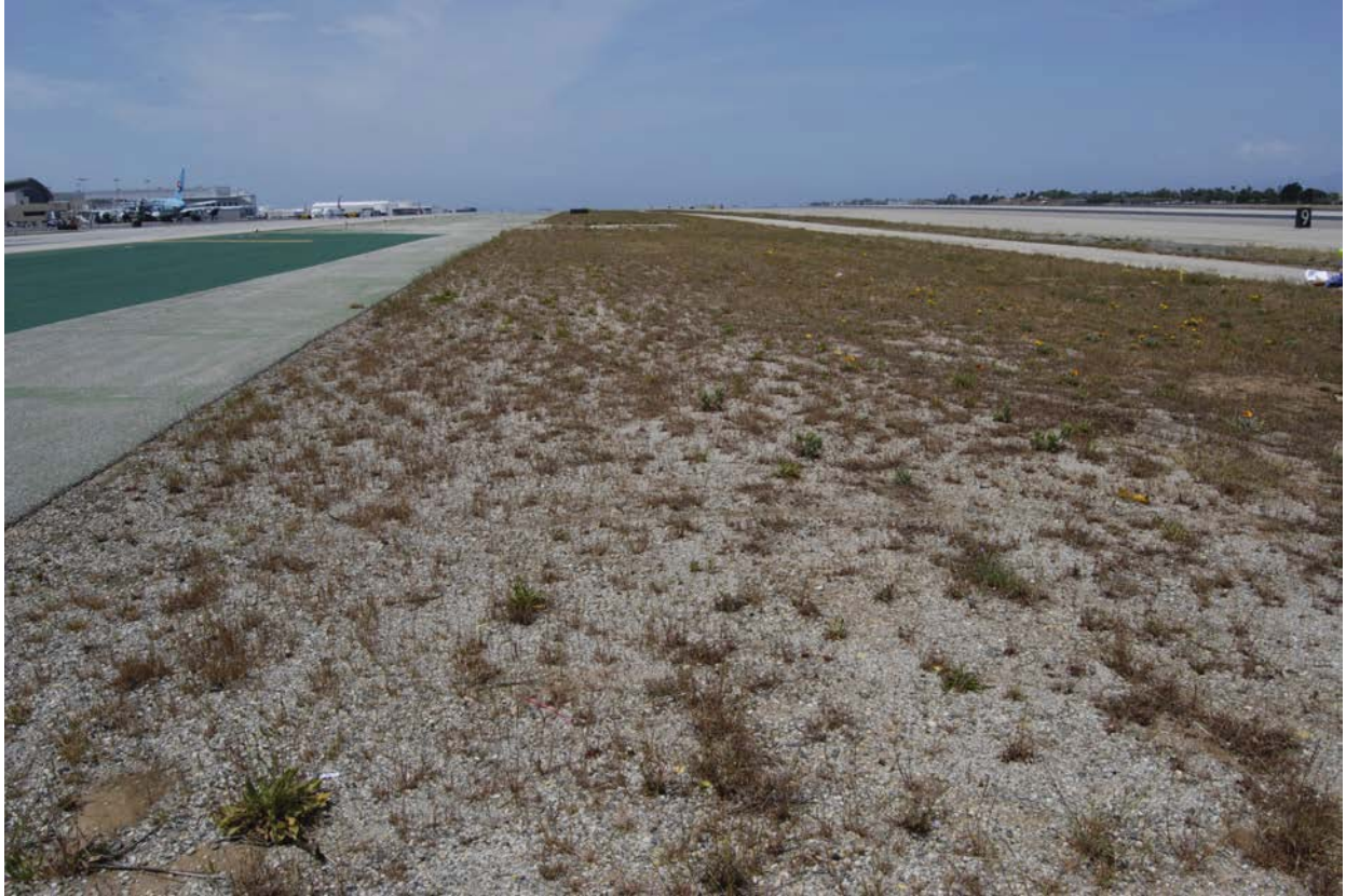
Image 5.2.1-5. Runway 6L-24R, facing west
