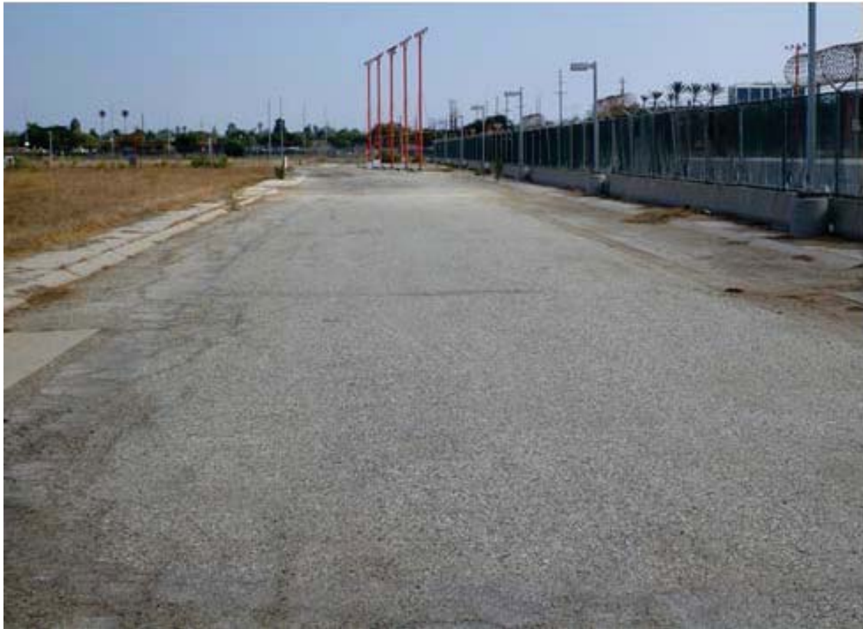
Image 5.2.1-4. El Manor Avenue, looking north
