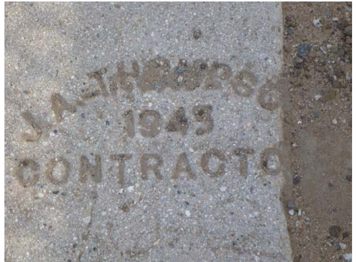
Sidewalk construction mark: closeup
