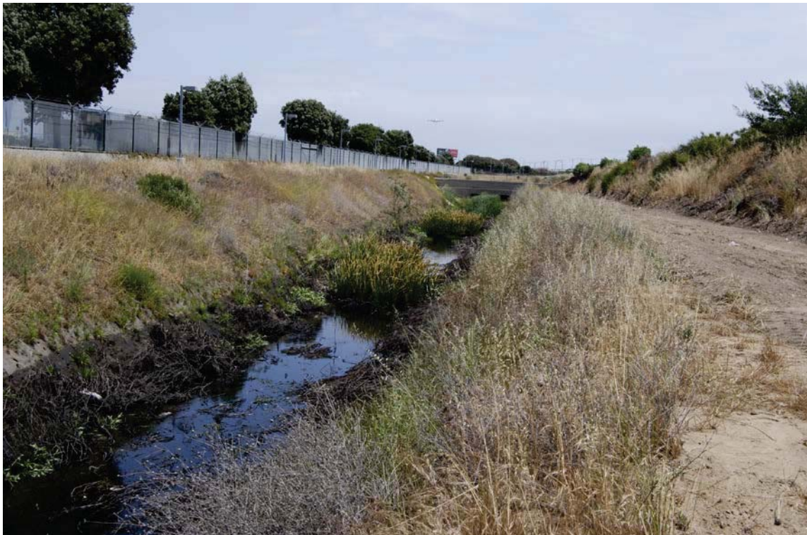
Image 2.2-2. Argo Ditch, facing northeast
