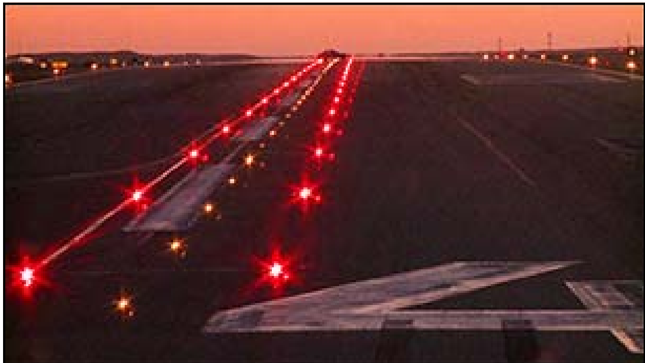
b. Existing North Airfield Runway 24L (Looking West ) In-Pavement Approach Light System, Similar to Proposed Runway 7L In-Pavement Approach Light System.
