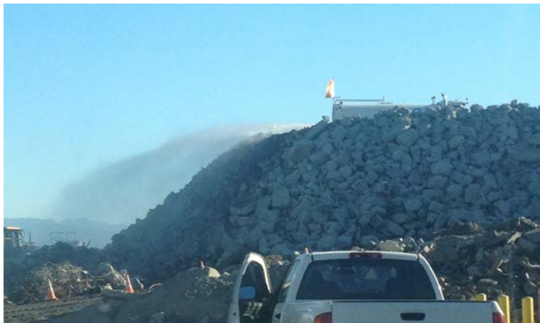
Water truck up top spraying the pile with water to prevent fugitive dust during the concrete crushing operation
