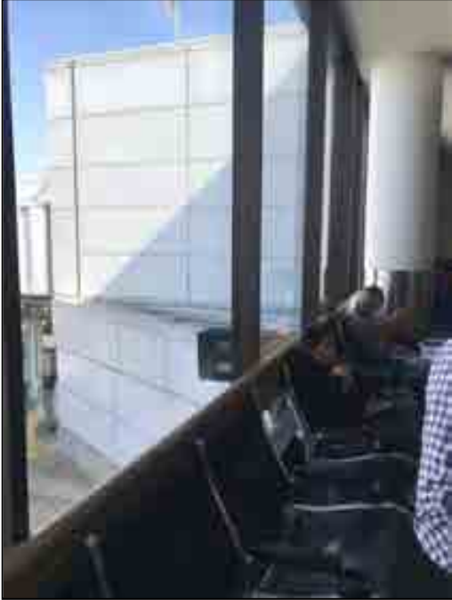
Photograph 2. Detail view of Terminal 6 exterior cladding and windows, October 7, 2019
