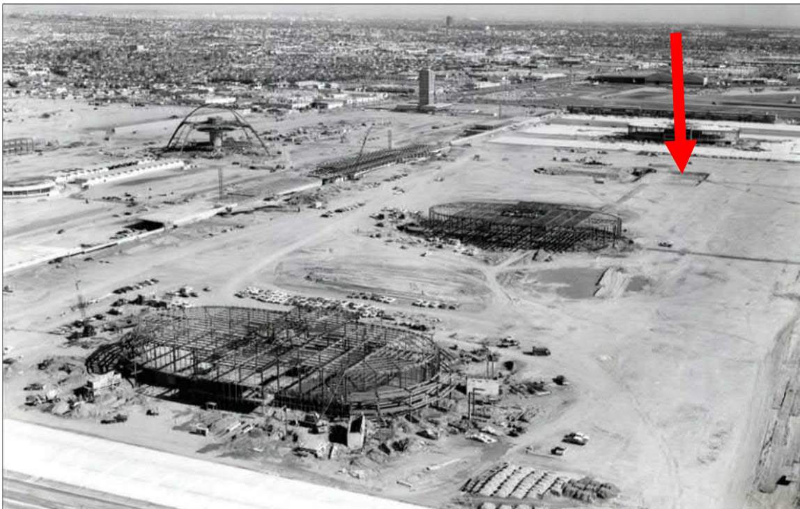
Plate 1. Beginning of construction for satellite Terminal 6 in 1960 (LAX Photo Archives 1960).
