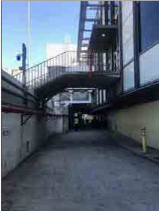
Photograph 4. View of Terminal 6 tunnel, October 7, 2019
