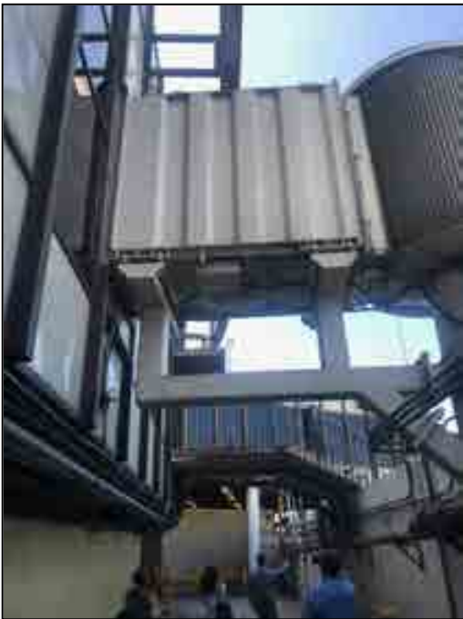
Photograph 3. View of passenger gate and windows from tunnel, October 7, 2019
