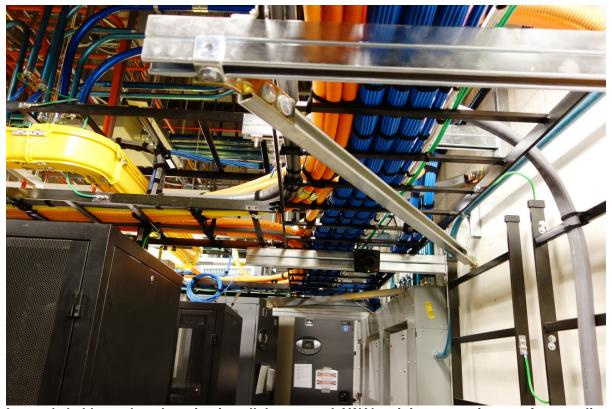
A sample ladder rack and routing install that meets LAWA's minimum requirement for a quality.
