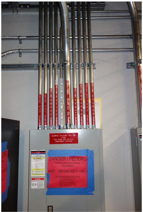
Sample electrical conduit and panel labeling.
