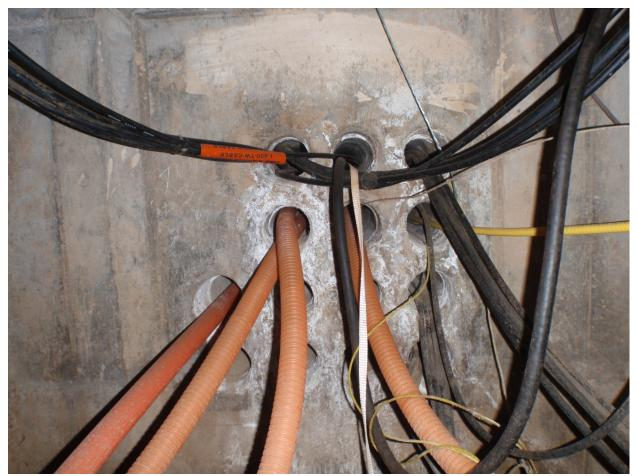
A legacy MH showing empty conduits without duct plugs and inflatable cable wraps leak.
