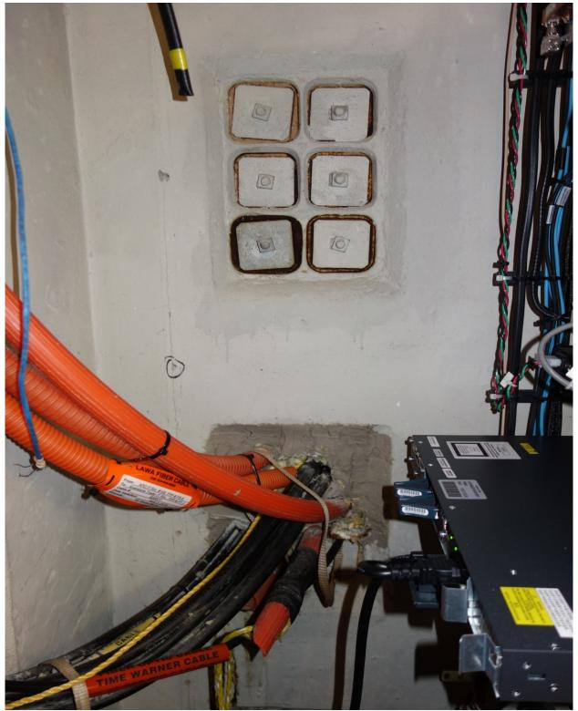
A legacy Maintenance Hole with a wall that is shared with a basement is prone to leaks.
