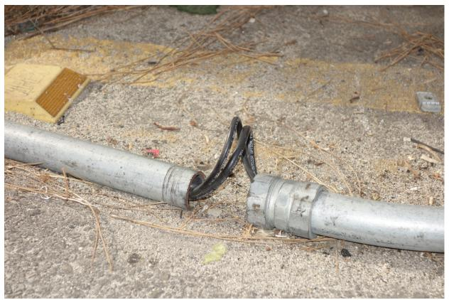
A sample of a rigid conduit coupling that has opened due to a lack of protection.
