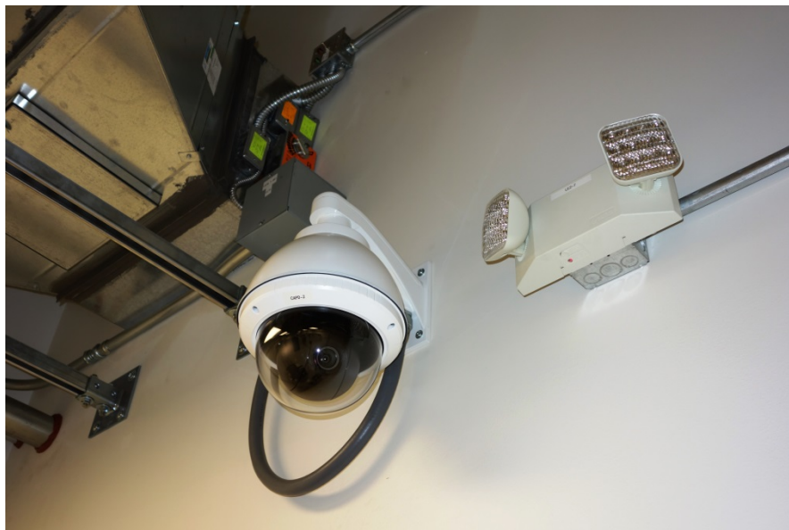
Sample Pan/Tilt/Zoom camera now used in IT rooms to replace Netbotz cameras.
