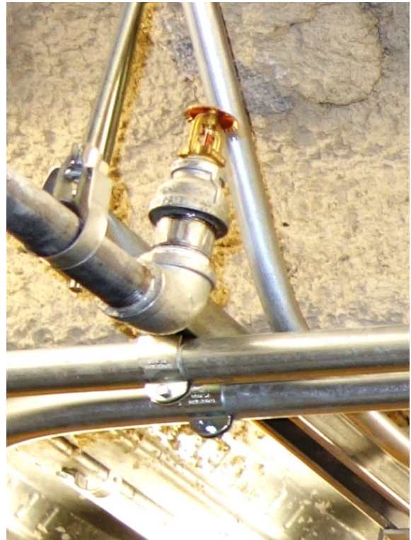
Sample IT Room sprinkler heads.
