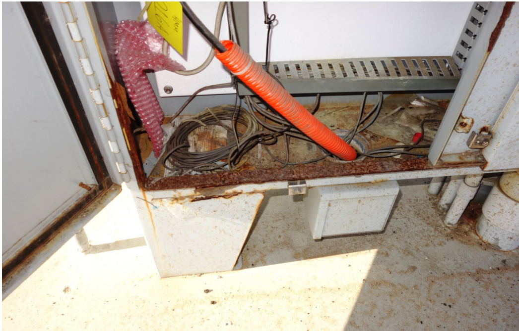
Rust is the reason for requiring outdoor TE's to be stainless steel.
