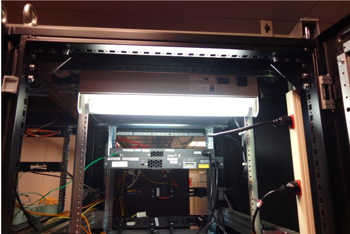
Cabinet light fixture can mount on the top.
