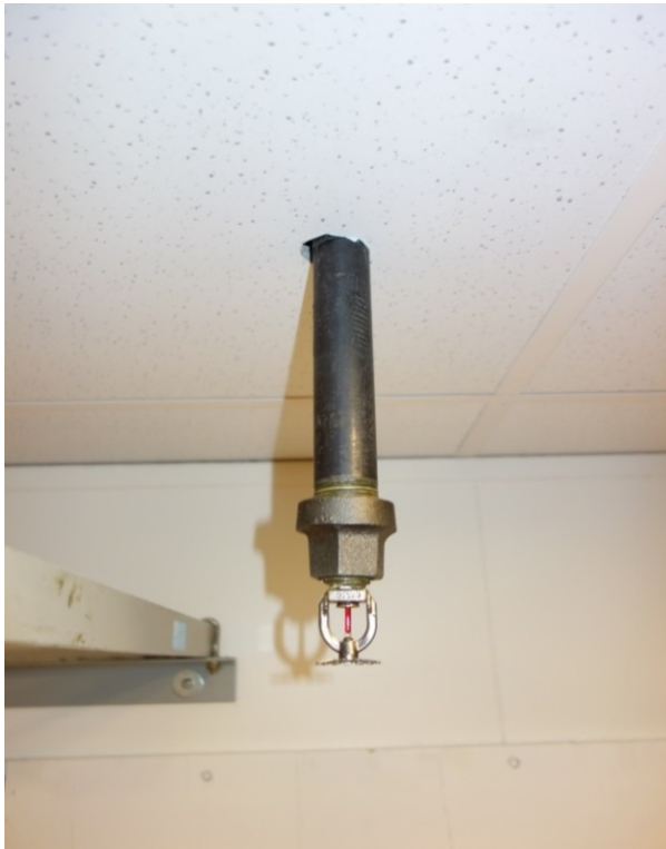
Sample IT Room sprinkler heads.
