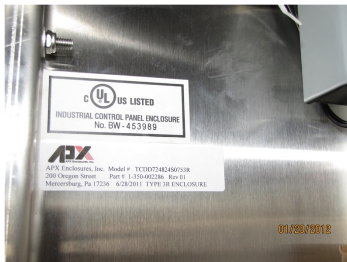
All TE's shall be UL listed and stamped.
