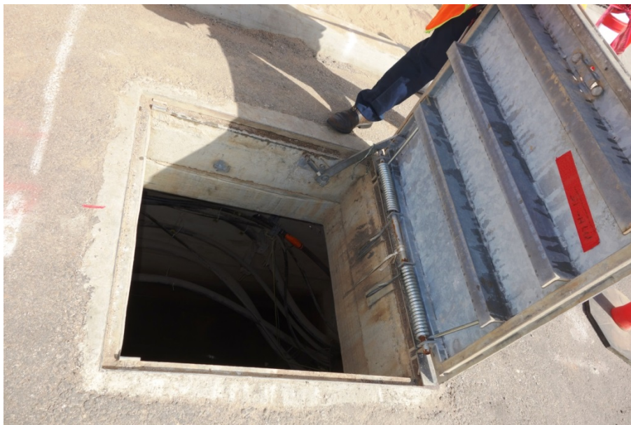
Maintenance Hole with a square cover and torsion spring assisted opening.
