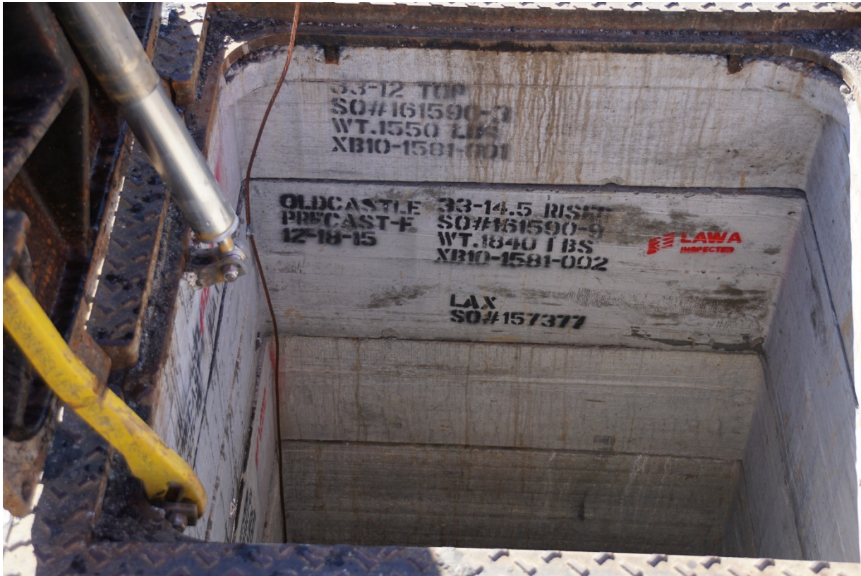
Deeper Maintenance Holes may need to be built up using pre-casted sections as shown here.
