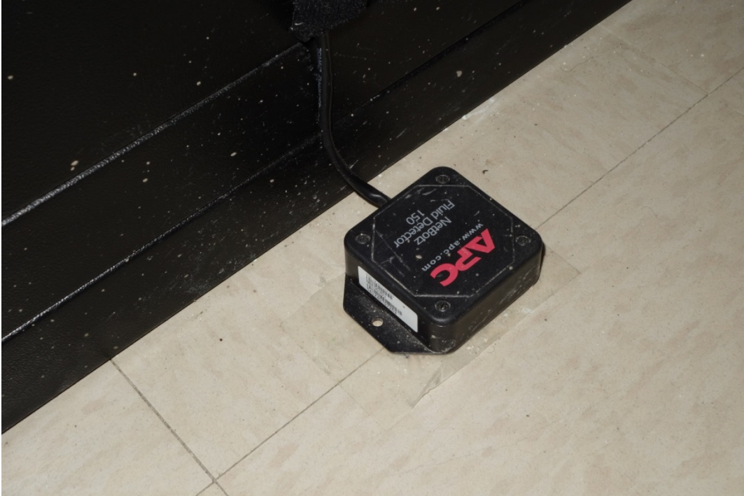
Sample Netbotz floor-mounted flooding sensor.
