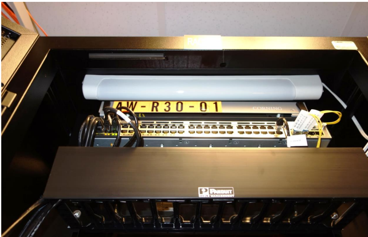
Cabinet light fixture can mount on the top – different fixture.
