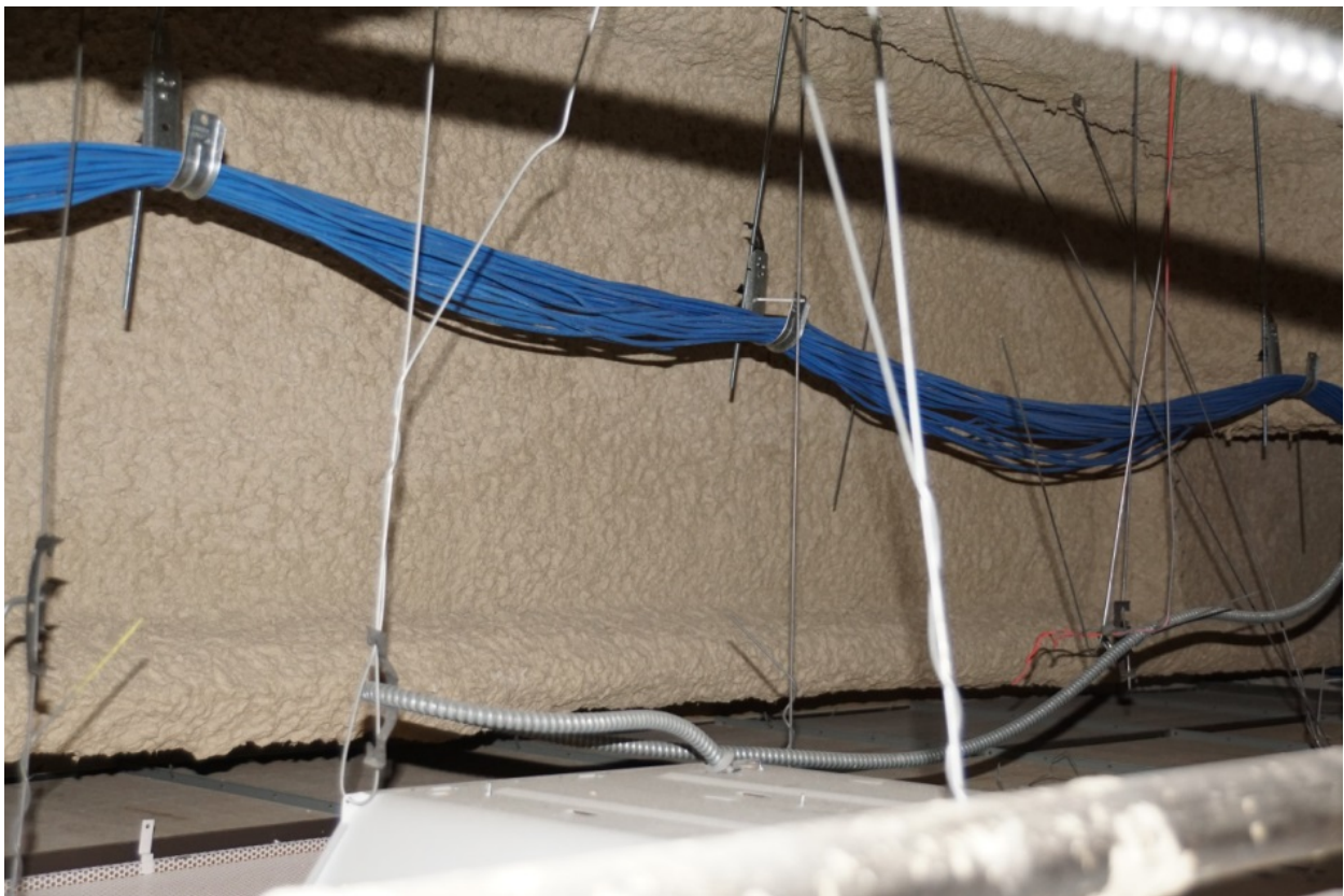
A simple J-Hook installation is shown.
