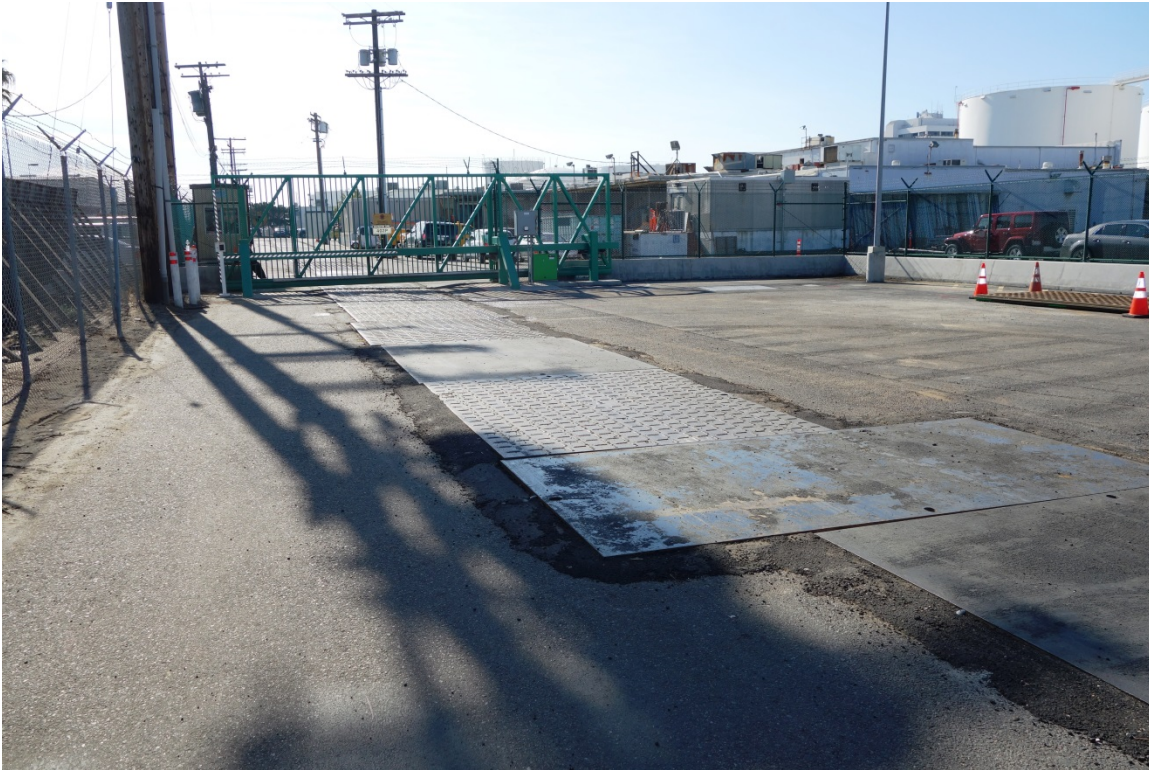
An open trench protected with steel plates asphalted in place.
