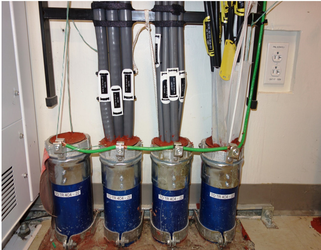
Conduit stub-ups shown secured to floor-mounted strut.
