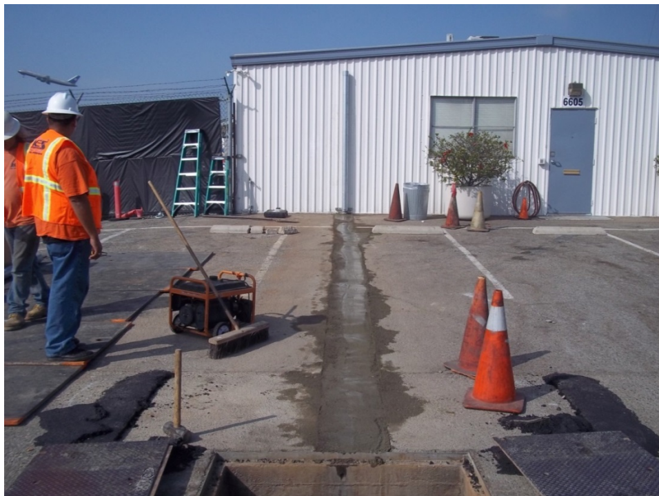
The finished trench matches the existing landscape.
