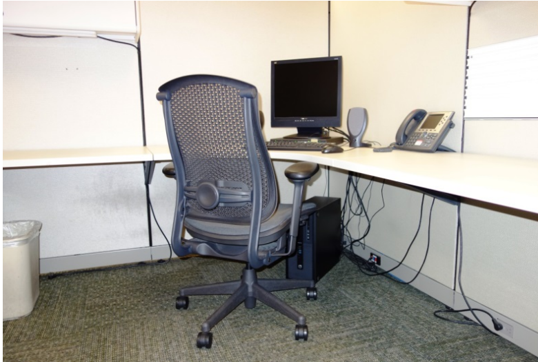
The standard cubicle is fed with two CAT 6 cables.
