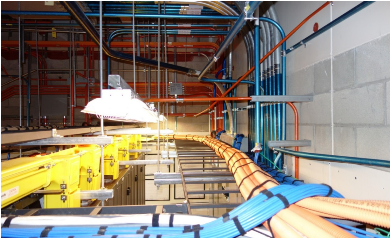
Cable Trays shall have neat combed cable bundles & straight cable lines.
