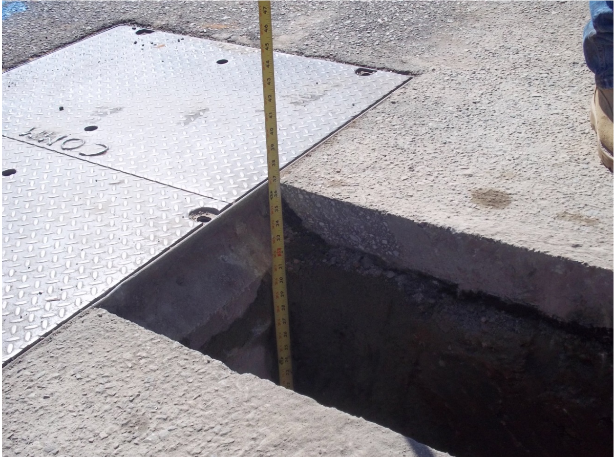
Trench depth per the National Electric Code.
