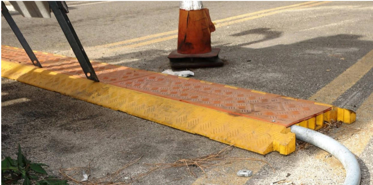
Conduit-protector in driveway protecting conduit.
