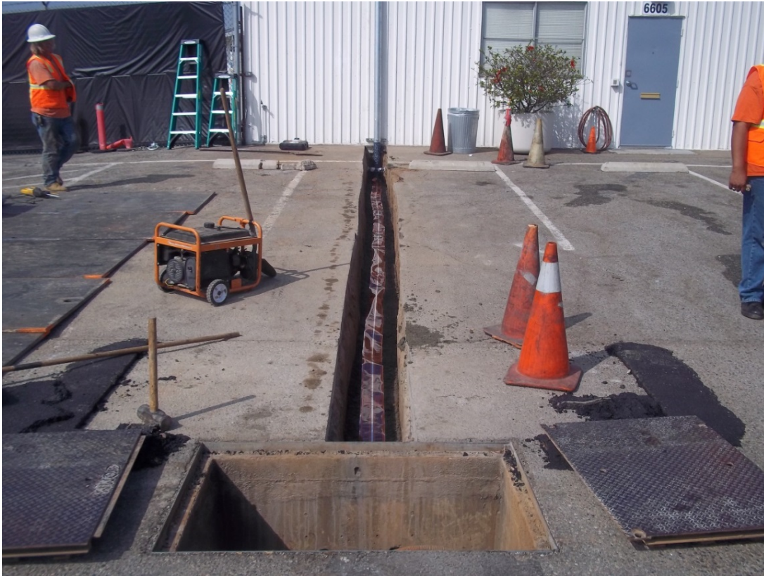
Underground detectable identification tape installed.
