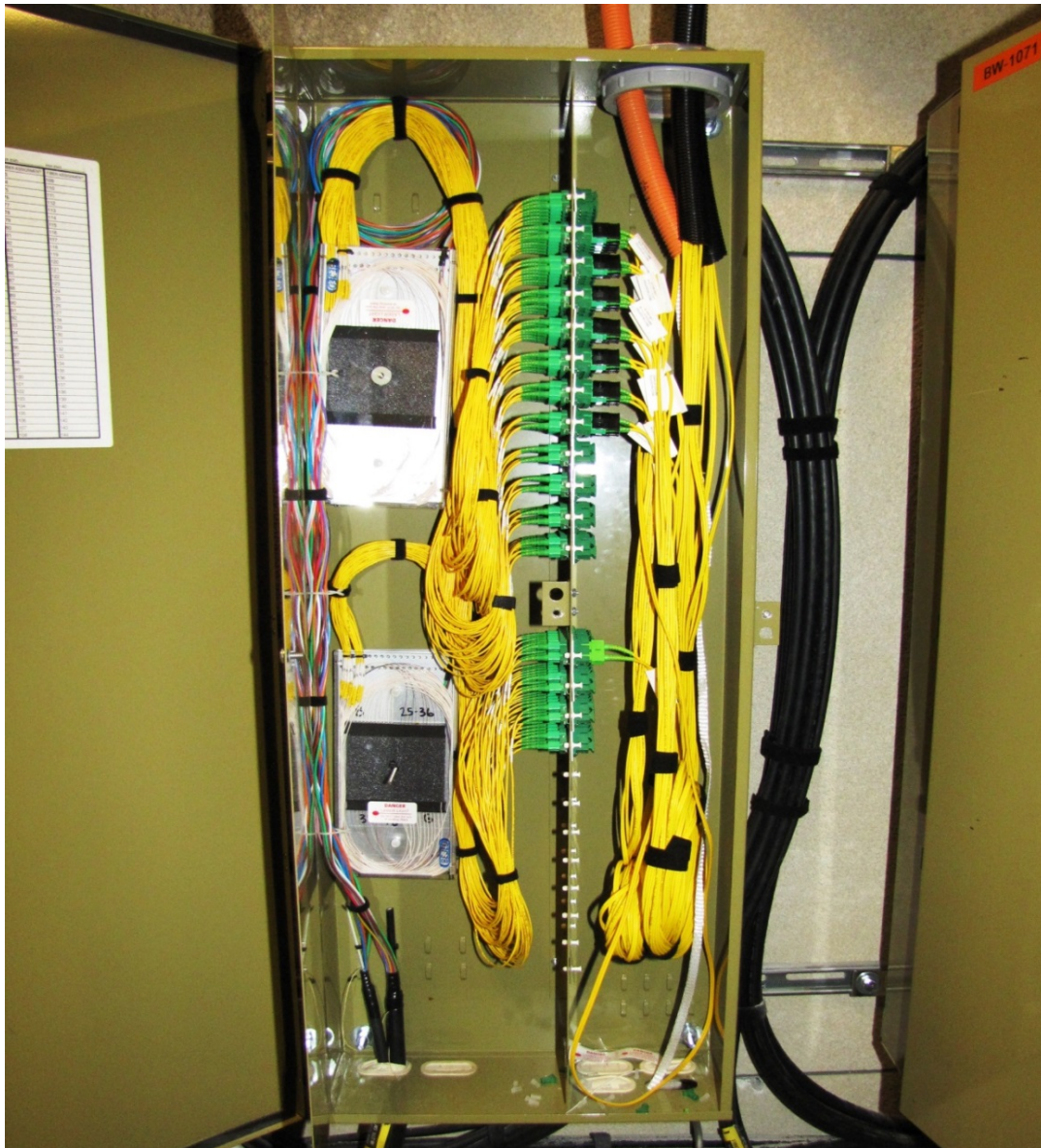
Splice trays are stacked, jumpers are labeled and less than 3 feet long.
