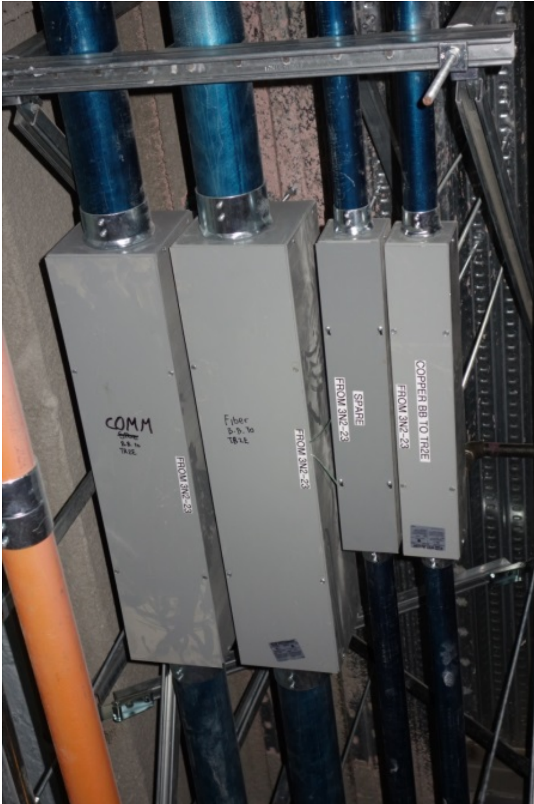
Pull boxes on straight runs for long cable pulls.
