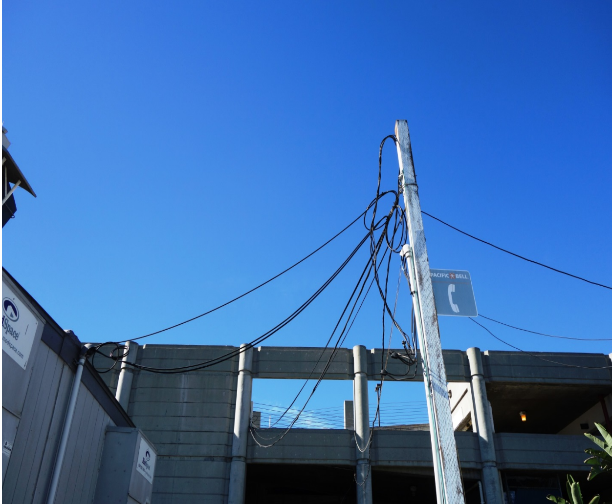
A temporary pole set up for a project trailer is shown.
