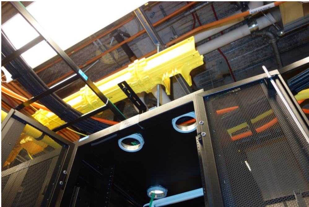
Fiber Trough shall not be used because of the difficulty aligning with cabinet chase nipples.
