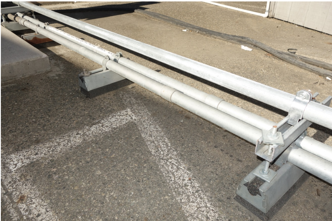
Asphalt support conduit pathway.
