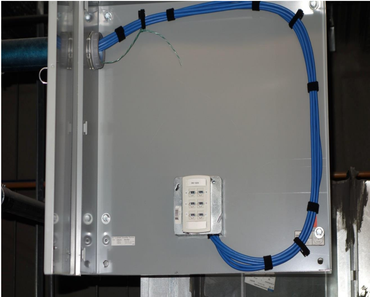
Consolidations Points may be as simple as a WOA in a 4S box.
