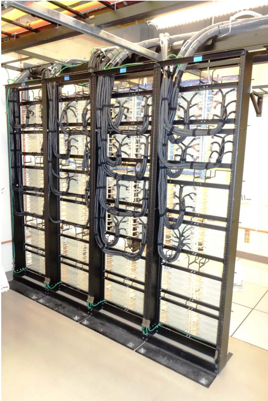
Rear View of an MPOE MDF shown with racks of 110 Blocks for Copper BD.
