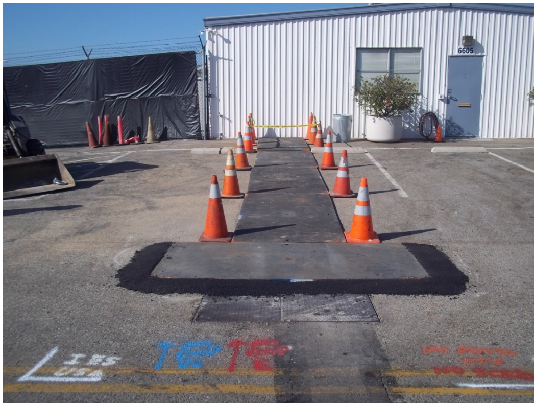
An open trench protected with steel plates asphalted in place.
