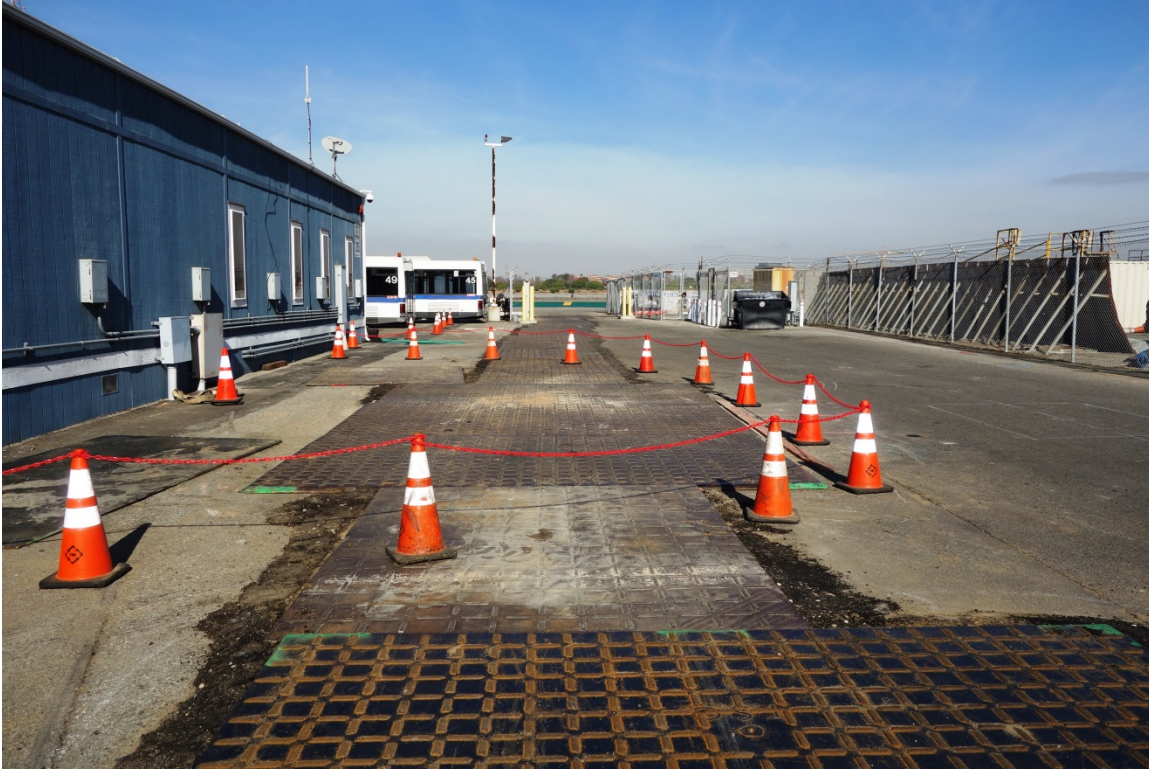
An open trench delineated with orange cones.
