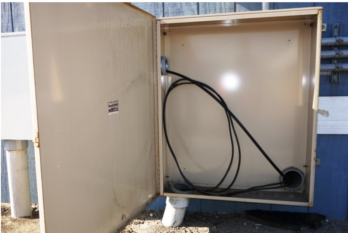
Outdoor pull boxes that are 24-inches square or greater shall have piano-hinge covers.
