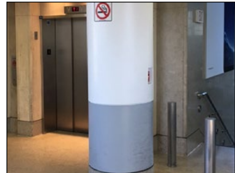
COLUMN ON PEDESTRIAN BRIDGE PREMESSAGING
