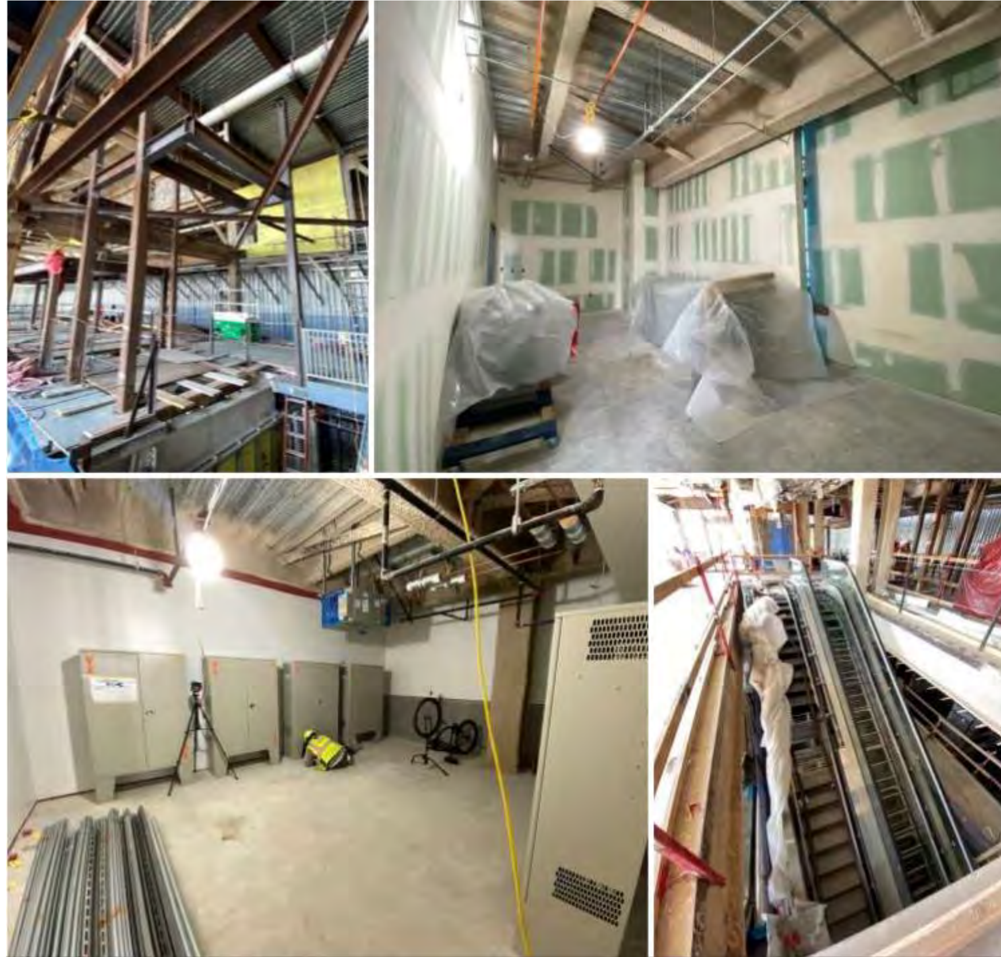
Area 2 – Roof Deck poured; Elevator/Esc Steel Installation; Interior Framing/Drywall; Piping and Conduit Installation
