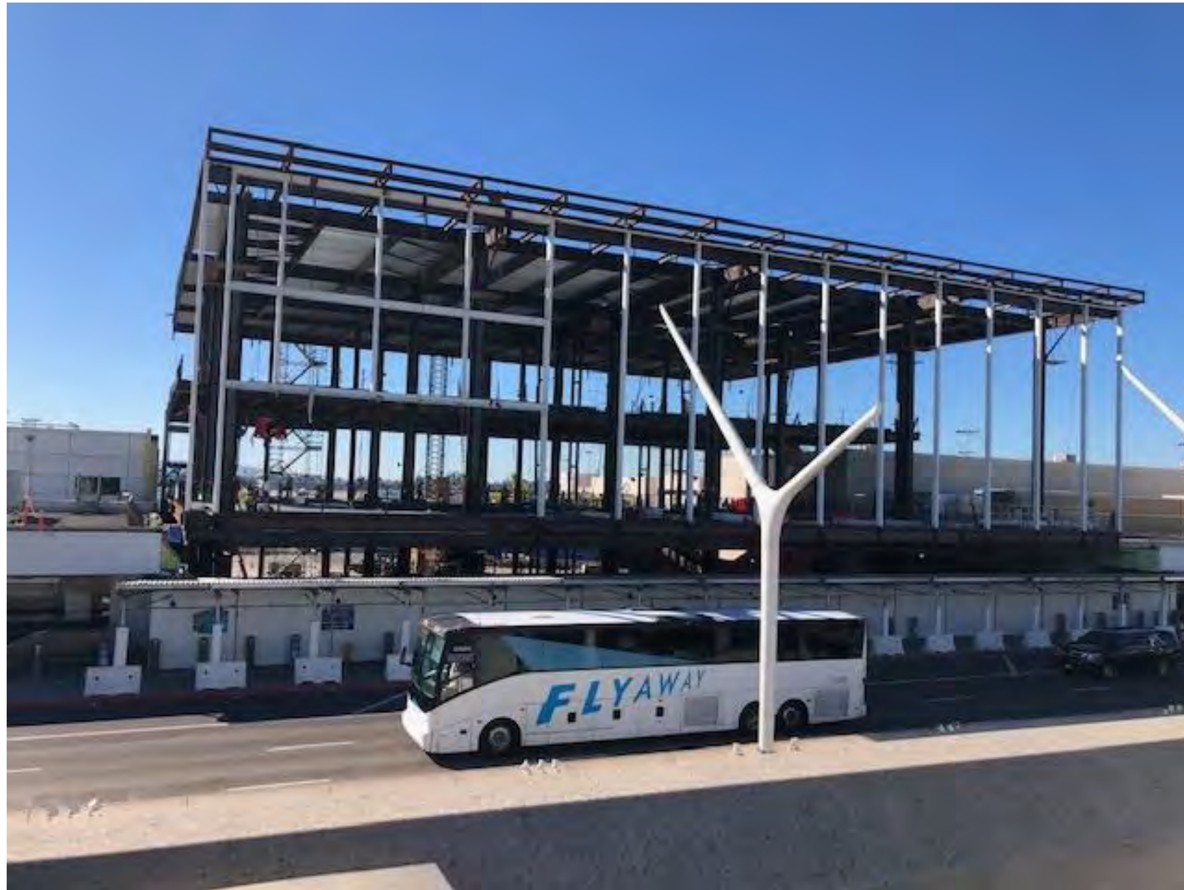
Looking South from CTA – steel erection complete; exterior skin will be installed in May 2021
