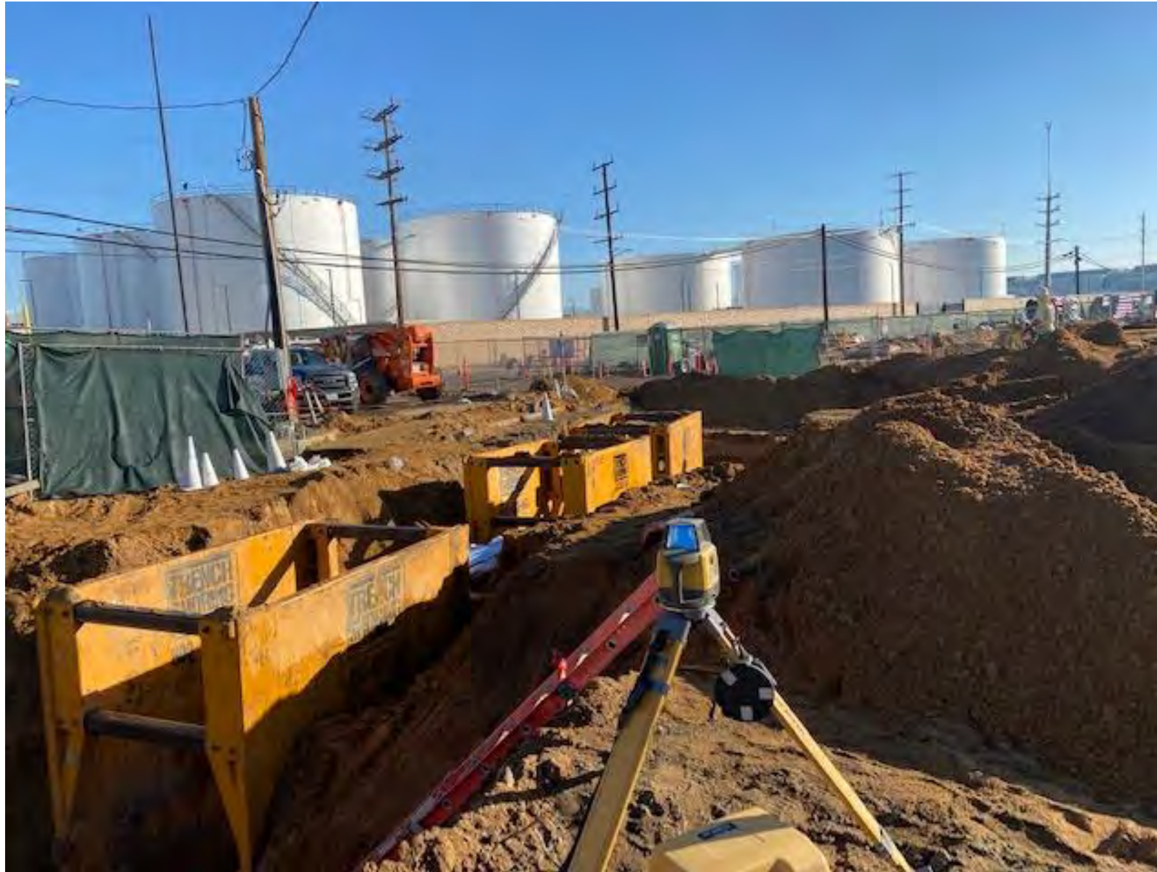
Building Demo complete; Trench/Shoring work in progress
