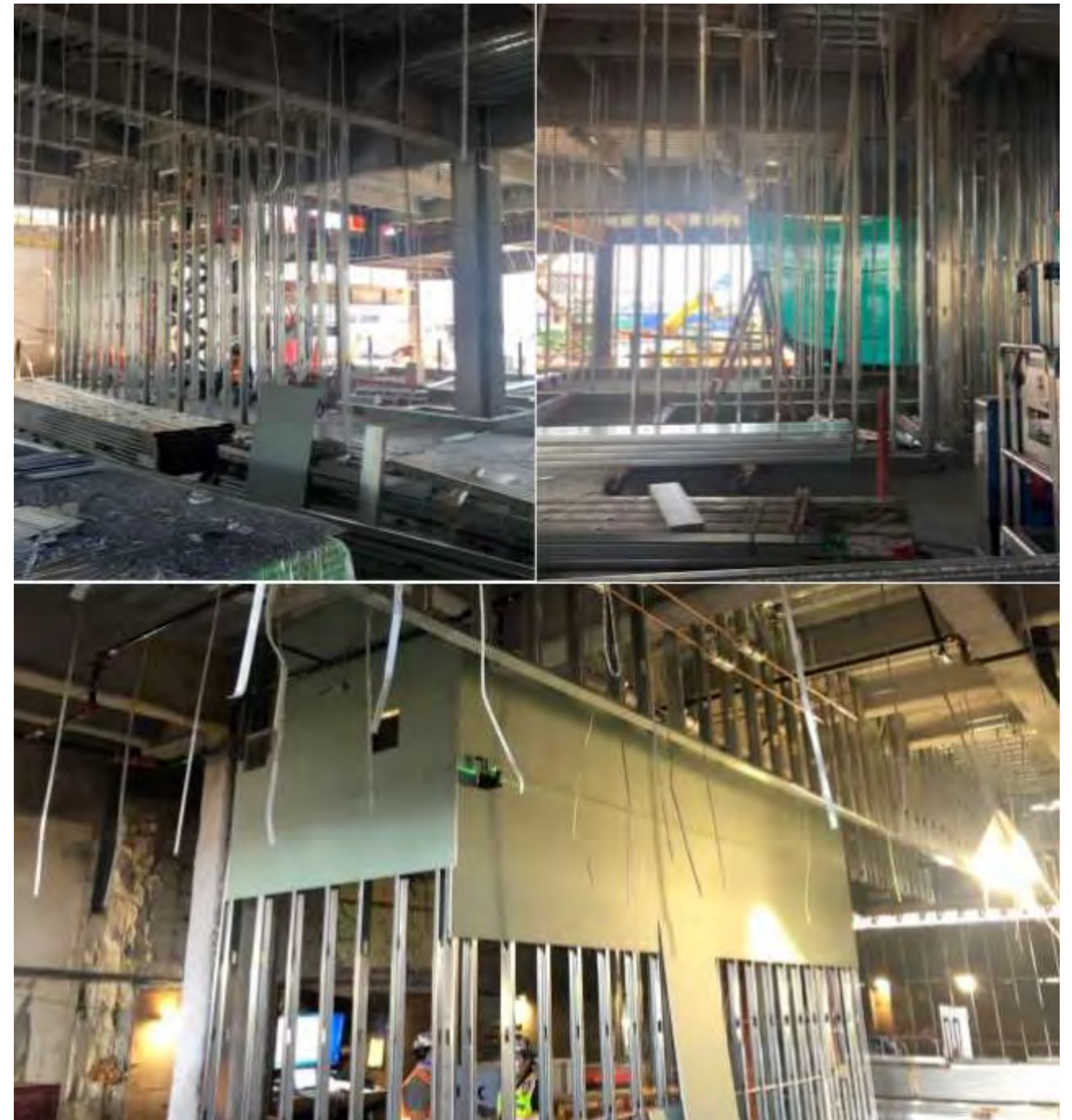
Layout of Interior Walls and Framing on all Levels
