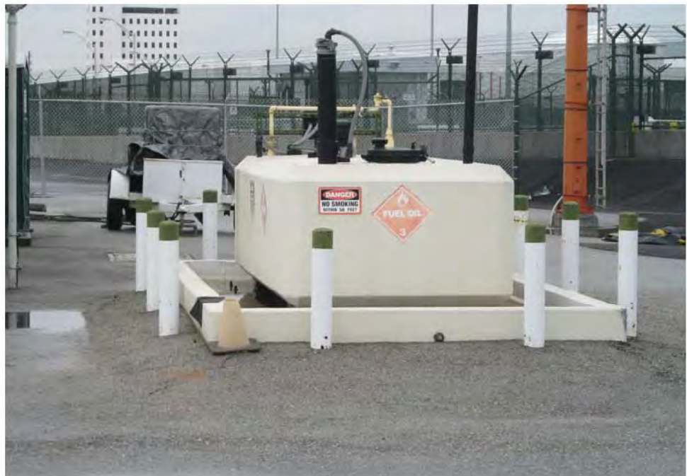
Photograph 80: View of 500-gallon diesel AST with secondary containment for an emergency back-up generator northeast of the FAA receiver/transmitter station building.
