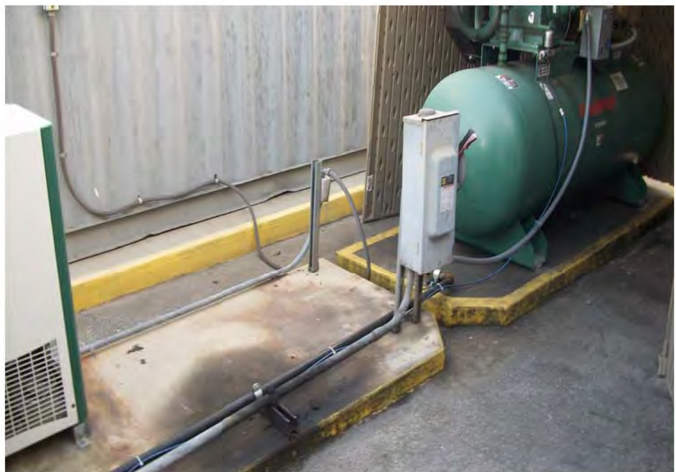
Photograph 18: View of air compressor and surface staining outside the northwest portion of the USCG Air Station.
