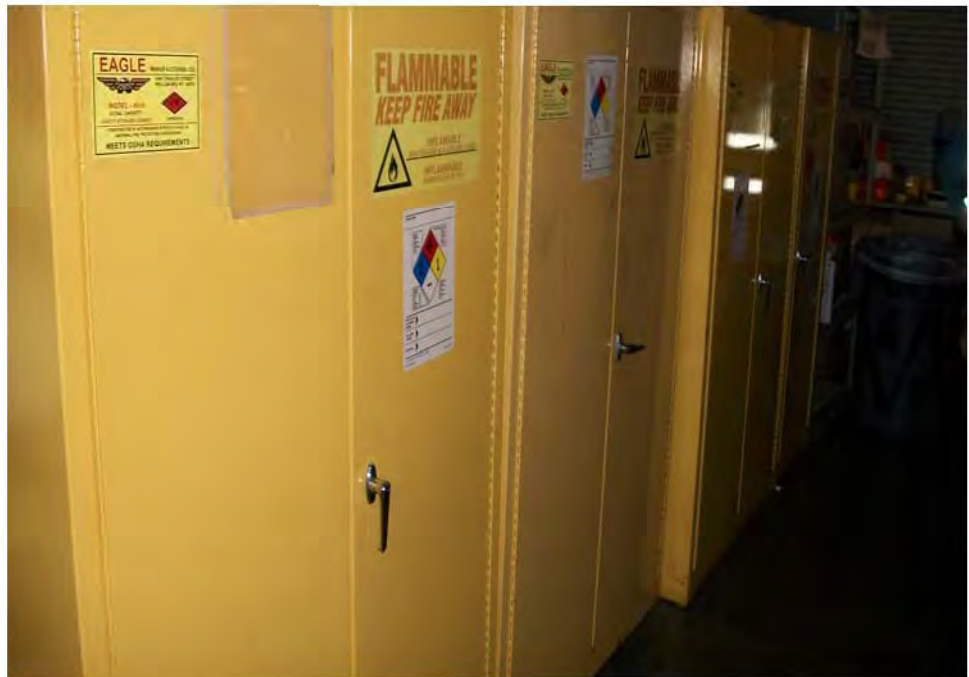
Photograph 53: View of fire cabinets containing small amounts of grease paint, solvents and adhesives within the in-flight storage area in the center of the Qantas hangar.
