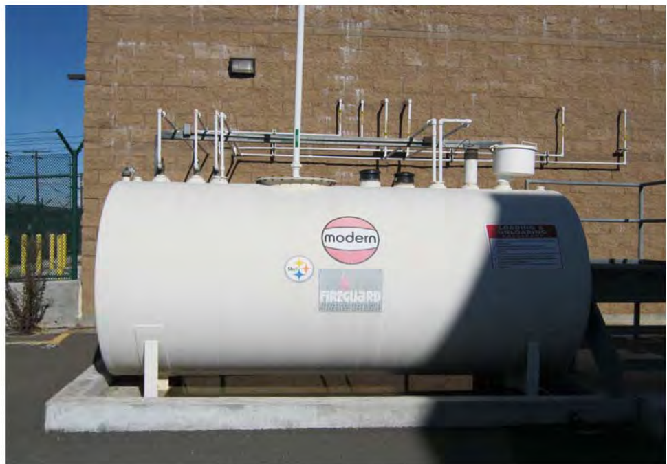
Photograph 26: View of 2,000-gallon diesel oil AST outside the southern portion of the electrical vault building.
