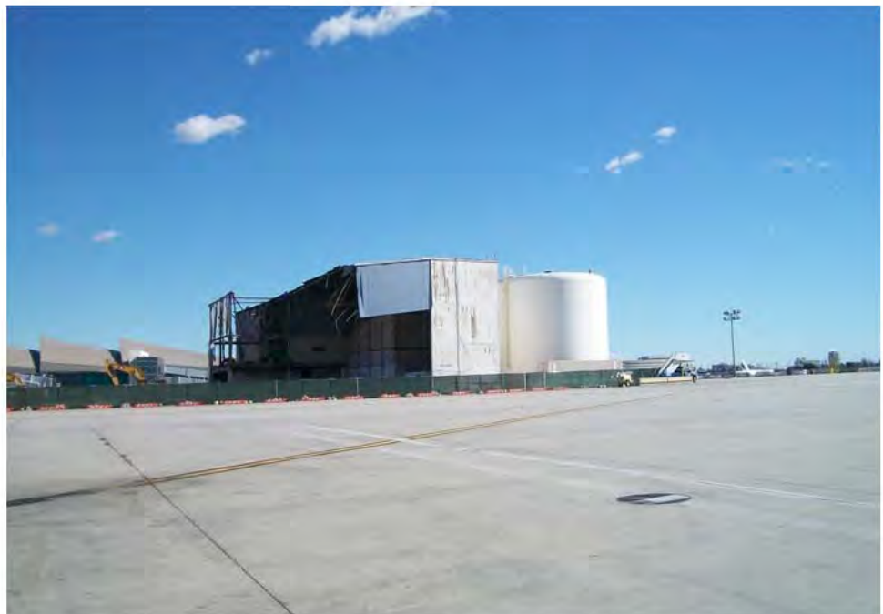
Photograph 102: Looking southeast away from the American Airlines hangar at former hangar with associated three 750,000-gallon empty water ASTs, currently being demolished.
