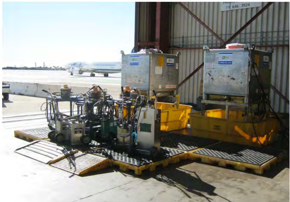
Photograph 90: View of engine oil ASTs with secondary containment in the southwestern portion of the American Airlines hangar.
