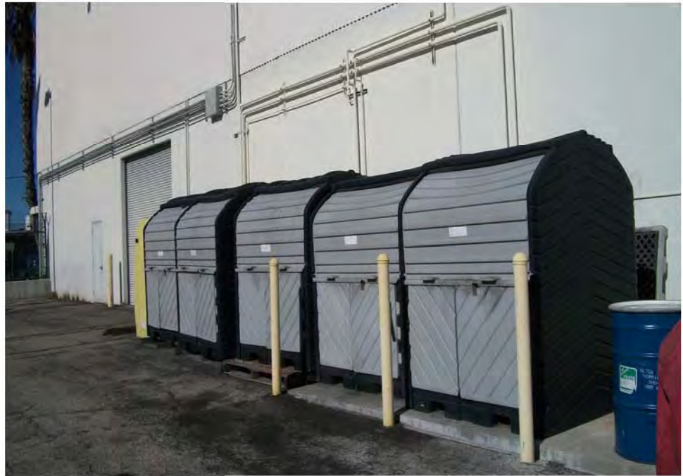
Photograph 45: View of waste oil drum storage containers containing oil filters, engine oil, and hydraulic fluid.
