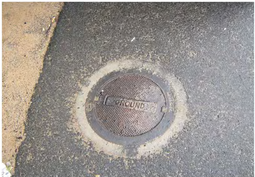
Photograph 32: View of one of the "Ground" wells that surround the electrical vault building.
