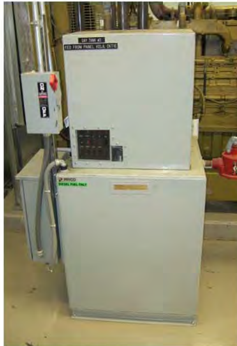
Photograph 31: View of 50-gallon diesel AST (bottom) and control panel (top) associated with back-up generator.
