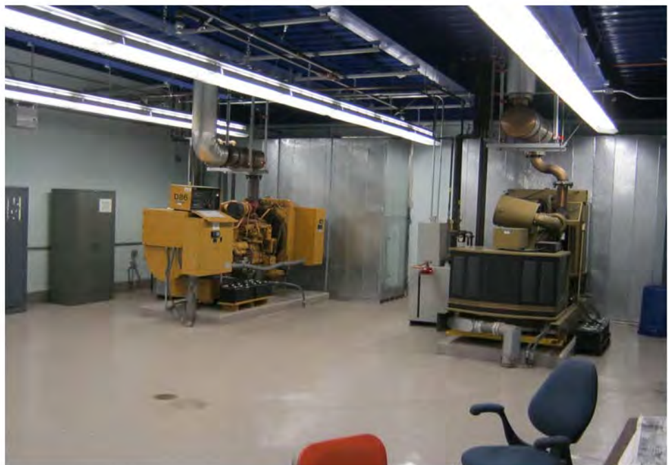
Photograph 30: View of back-up generators in the southern portion of the electrical vault building.
