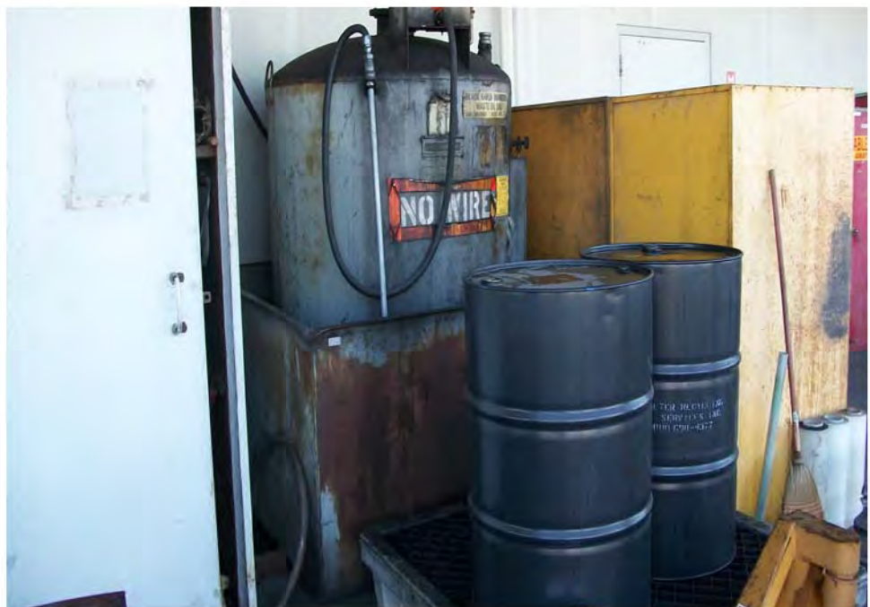
Photograph 34: View of 500-gallon waste oil AST and two 55-gallon waste oil drums outside northern portion of US Airways hangar.
