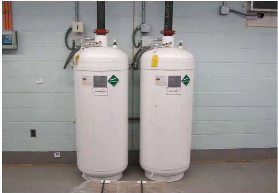
Photograph 29: View of pentafluoroethane storage tanks for fire suppression in electrical vault building.
